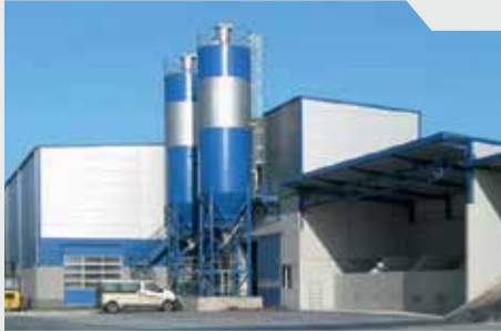
Concrete batching plant
